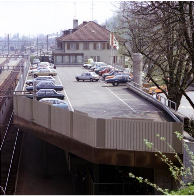
Station forecourt in Switzerland: Ice and snow don't have a chance in the heated parking lot
