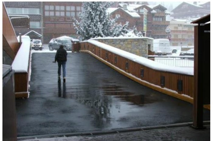
Heated pedestrian bridge during snowfall: safety for the users
