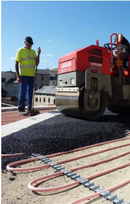
Installation of a MULTIBETON outdoor heating
