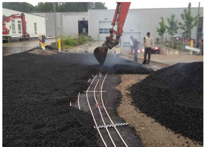
Nolte-Küchen, 2012, installed by company Busch GmbH & Co. KG in Bünde, Germany
