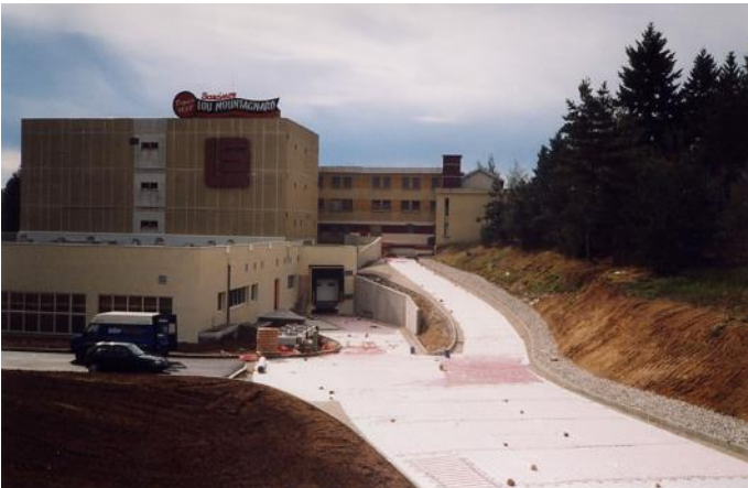
Private road of the brining "Les Montagnards " in Saint Maurice de Lignon / France, laid in 1999 by MB partner SABY , heated with waste heat from the cooling units of the brining
