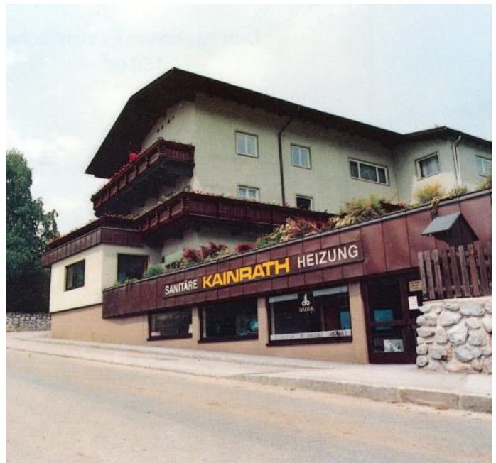
Sidewalk and parking lot heating, 1985, MB partner Kainrath in Jenbach, Austria
