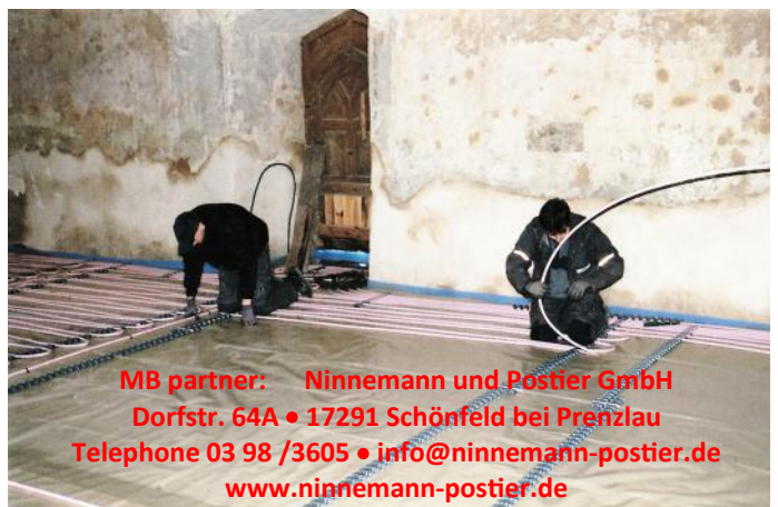
MULTIBETON underfloor heating being laid
